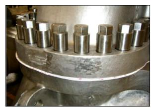
An analysis of the loading of the flange was completed and the proper gasket and bolt stresses were determined for a reliable seal. This resulted in a gasket recommendation of Teadit's 1/8" thick expanded PTFE style 24SH and flange assembly procedures including torque values and thread lubricant recommendation. The facility was unfamiliar with ePTFE material, and they wanted to perform a test to confirm that the soft material would not
